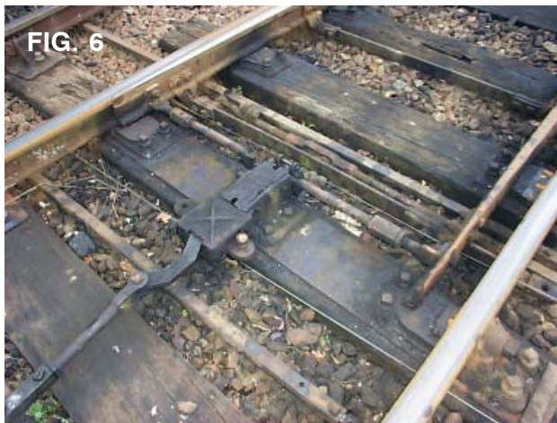
Fig. 6 There are three tie-bars on this A-switch. The second and third are reproducible in 4mm scale from the proprietary component packs, while the first tie bar and the facing point lock casting would need special sourcing as of 2008. The first slide chair timber takes a heavy side impact thrust as each wheelset rides onto the toe of the switch and is deflected suddenly to one side. It is a requirement on the prototype passenger lines to introduce a steel sole-plate beneath the slide chairs on timbered junctions so as to maintain gauge at the switch tips. The plate ensures that lateral forces are shared between all eight chair screws instead of just the outer four. It is reproducible in 4mm scale with 5-thou plastic sheet stuck to the upper surface of the timber to represent the plate, with 10-thou pieces secured with solvent to the outer edges to represent the ribs. The ribs maintain the slide chairs in the correct place and maintain gauge.
